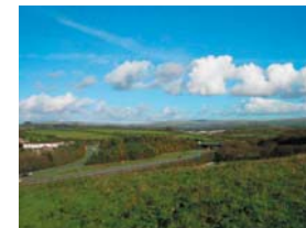
Dep Lane from South West
