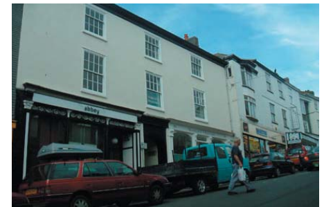
Kingsbridge High Street
