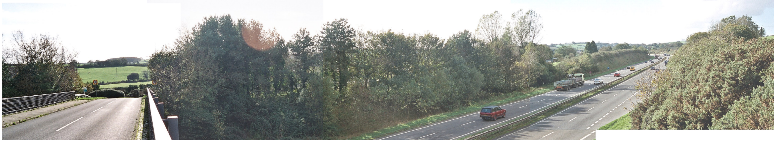
VP18 - A38 from flyover bridge near Lee Mill (existing baseline)
